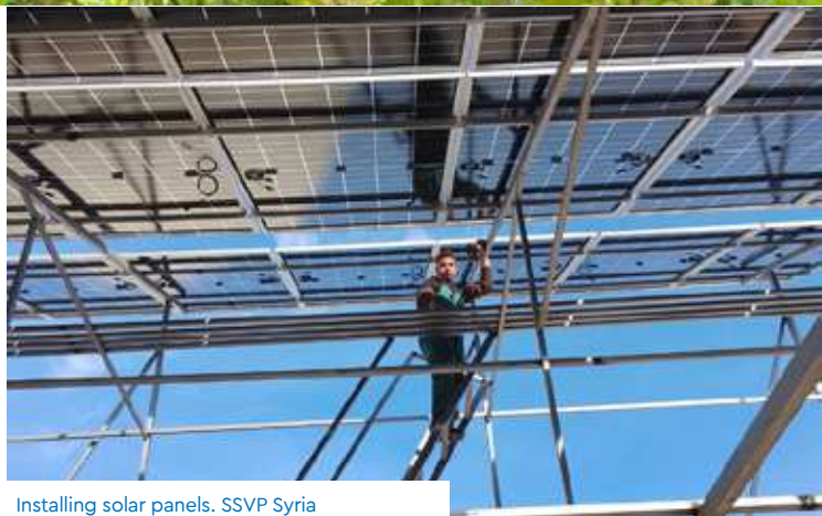
Installing solar panels. SSVP Syria
